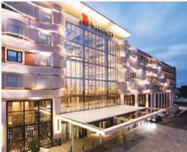
Marriott Auditorium Hotel, Madrid, Spain
