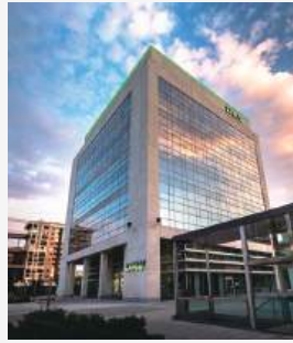
HQ Mansion of DKV, Spain
