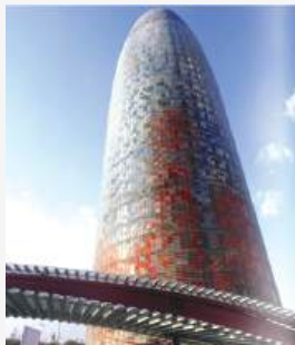
Torre Agbar, Barcelona, Spain
