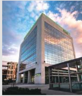
HQ Mansion of DKV, Spain
