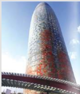
Torre Agbar, Barcelona, Spain
