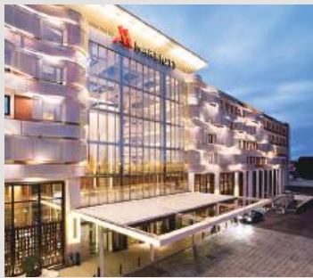
Marriott Auditorium Hotel, Madrid, Spain
