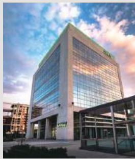
HQ Mansion of DKV, Spain
