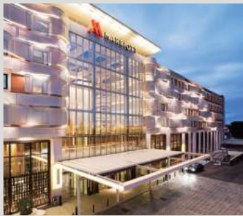
Marriott Auditorium Hotel, Madrid, Spain
