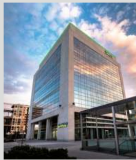
HQ Mansion of DKV, Spain
