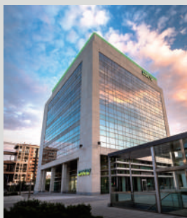
HQ Mansion of DKV, Spain
