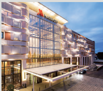
Marriott Auditorium Hotel, Madrid, Spain
