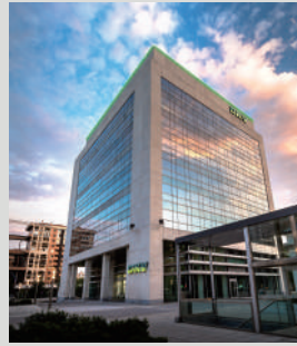
HQ Mansion of DKV, Spain
